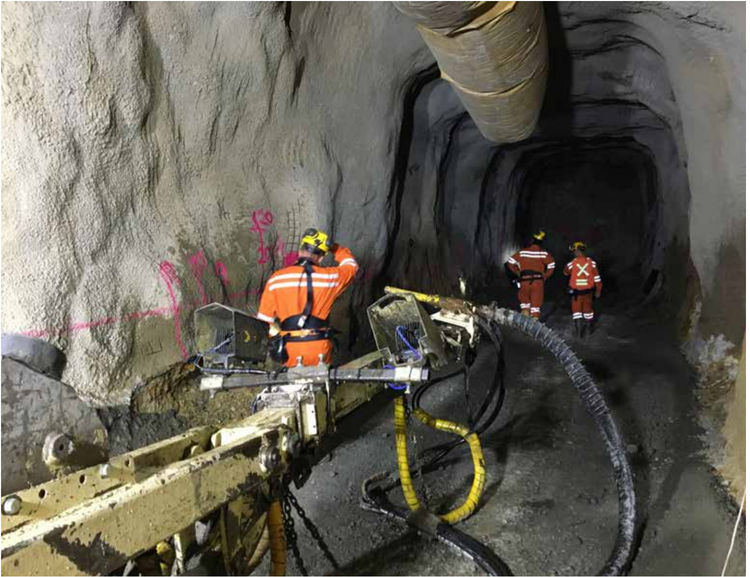
Shotcrete testing and shotcrete quality control underground.
