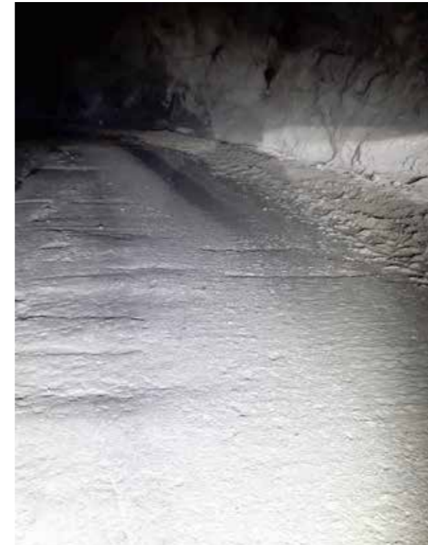
Concrete slabs along the main haulage ways of the mine.
