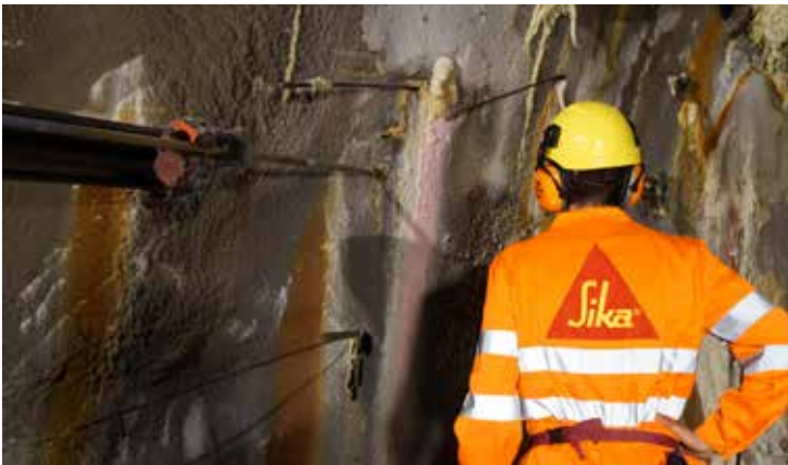
SikaFix® injections to counter water ingress underground.
