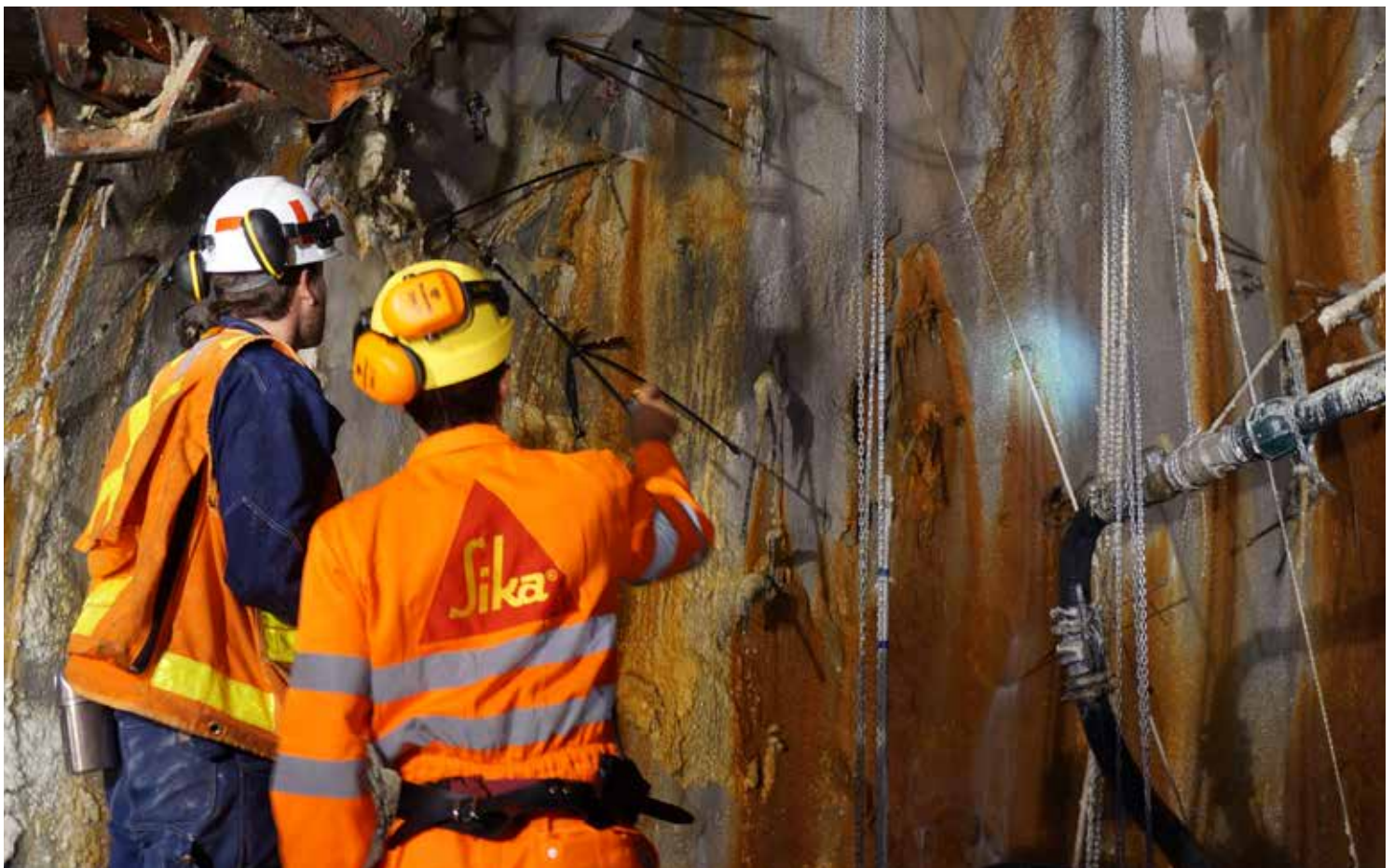
Observing the injected face with the stopped water ingress.
