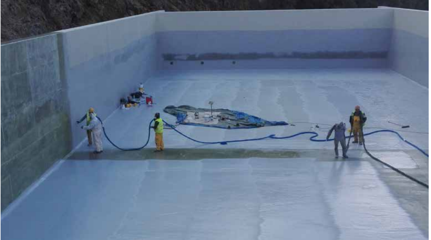
Spray application of Sikalastic®-843 GP using a two-component pump.
