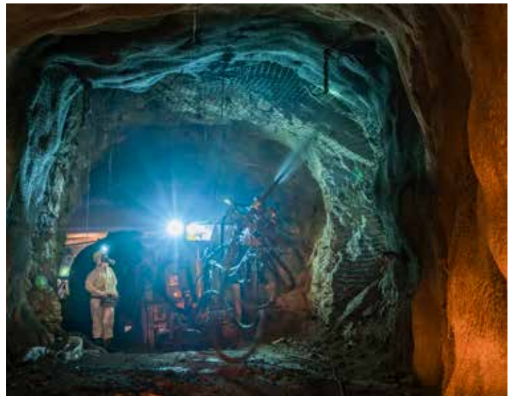
Shotcrete spray application using Sika® Sigunit® accelerator technology.
