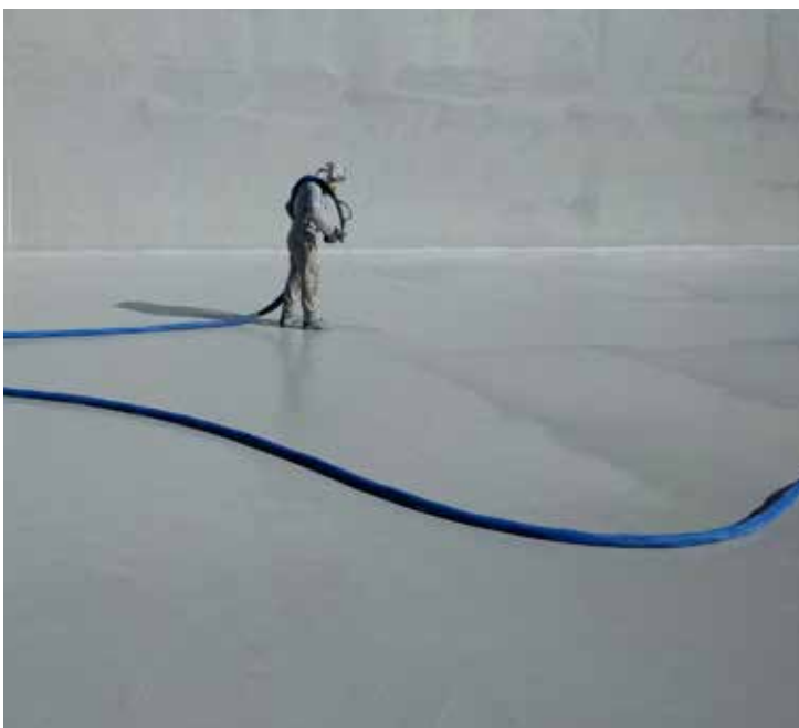
Spray application of Sikalastic®-843 GP in progress.
