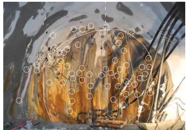
○ Unsuccessfully drilled injection holes prior to Sika injection process.
